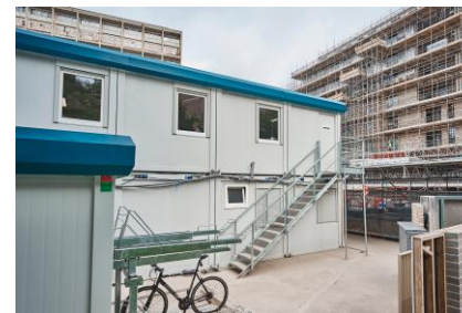
Construction site cabins
